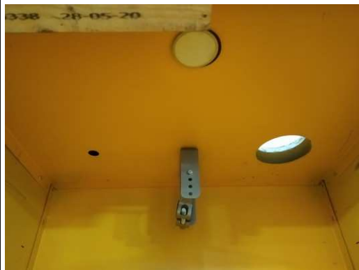
Hole for ventilator
