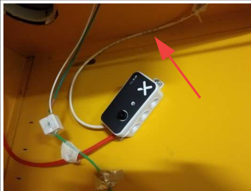
AF-X TEC Panel with linear heat detection (red arrow)
